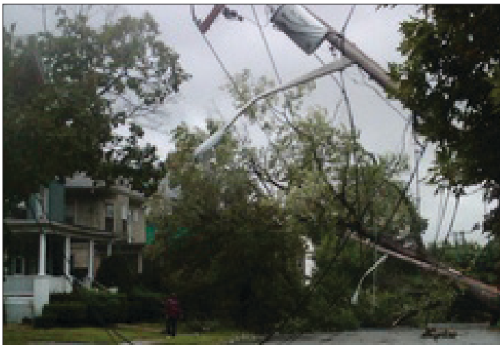
Power lines down from Irene
