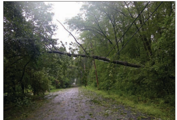
These lines were still live!
